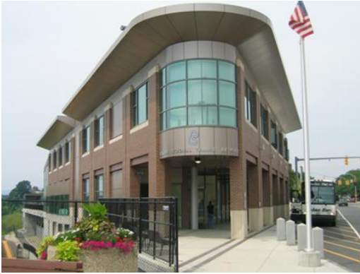
BRTA Intermodal Transit Center, One Columbus Avenue, Pittsfield, MA
